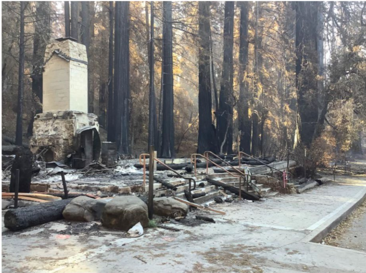
Figure 1. Administration Building, camera facing southeast. September 28, 2020.
