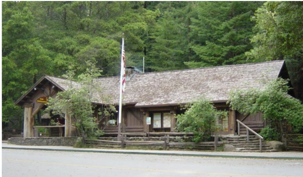
Figure 3. Administration Building, camera facing northeast. May 20, 2008.
